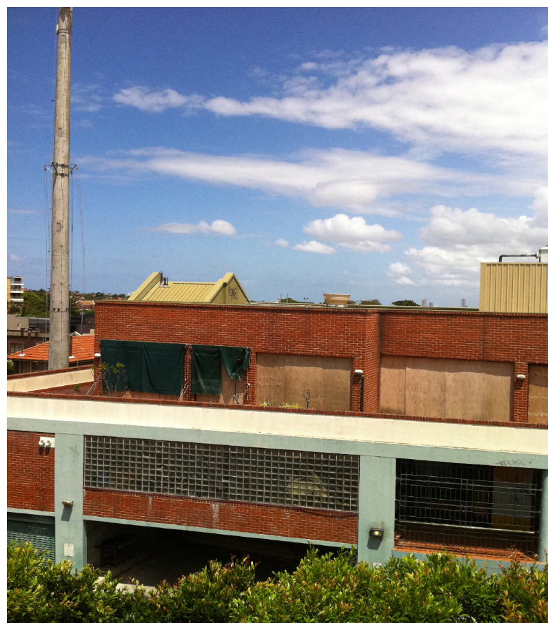
Figure 5: Standing view from the roof top terrace 16/5-9 Clifford Street
